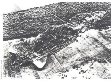
The Hindenburg disaster happened because the hull was filled with hydrogen gas. When mixed with air, hydrogen burns easily; one little spark would have been enough to set the whole airship alight. The designers knew that it was extremely dangerous to use hydrogen inside the airship. They had planned to use a new gas called helium which was much safer. But helium
